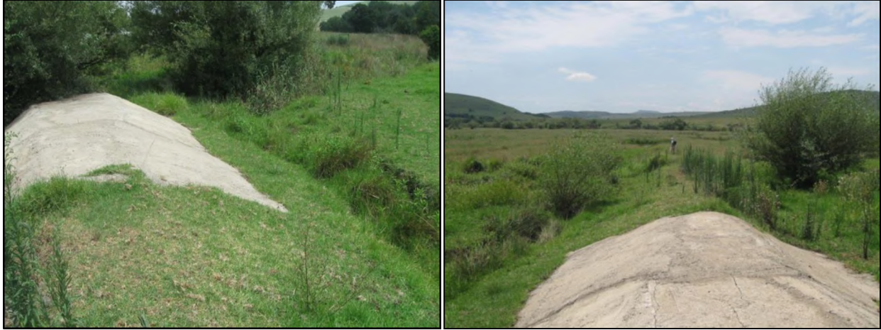
Plate 3.3. A concrete-covered earthen berm diverting flows out of the main channel in Kruisfontein wetland
