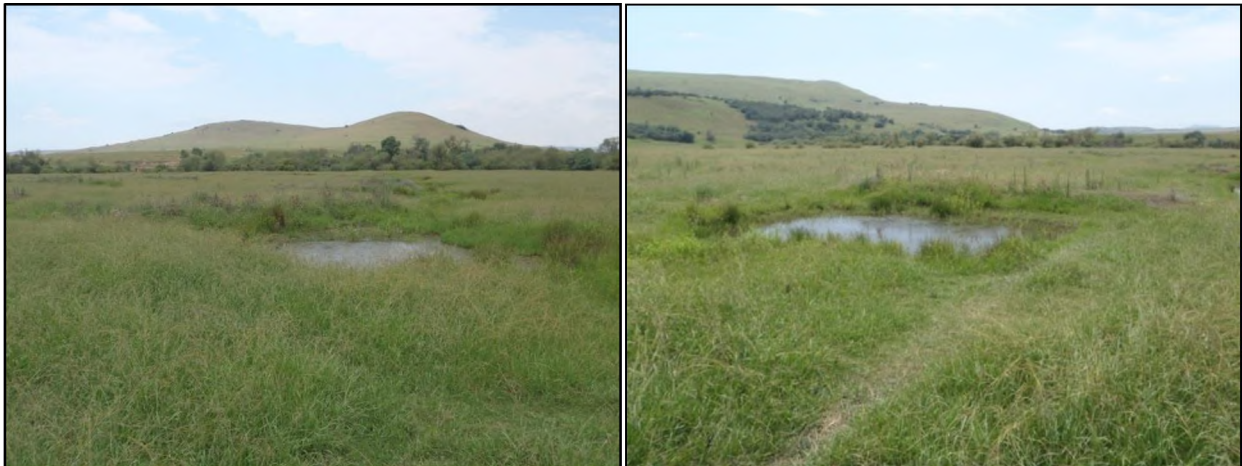
Plate 3.4. A series of earthen berms used to deactivate the ridge-and-furrow drainage in Kruisfontein wetland.
