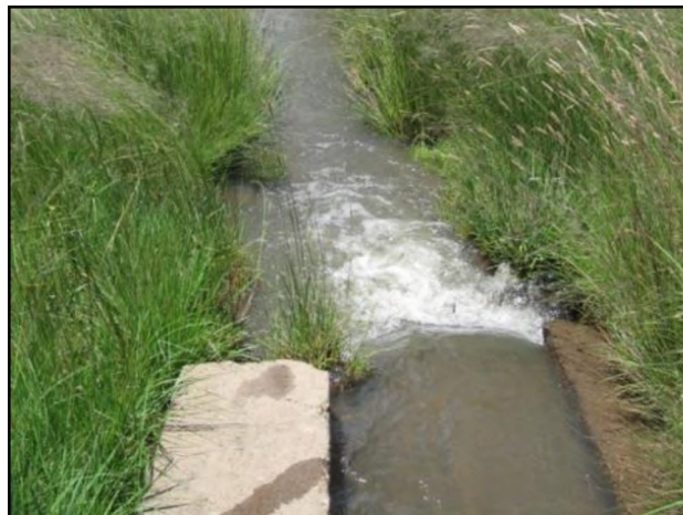
Plate 3.2. A spreader canal diverting a portion of the base flows out of the main channel in the Killarney wetland
