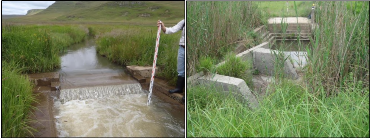
Plate 3.1. Concrete weir in the main channel of the Killarney (left) and Kruisfontein (right) wetlands.
