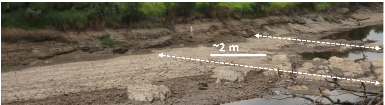
Plate 5.1. Photos of bedrock showing evidence of planing to a common elevation across the width of the river bed. The upper photograph was taken near Transect 9, at 90 masl, the middle photograph was at 85 masl, just downstream of Transect 10, and the bottom photograph corresponded with Transect 14, at 70 masl.
