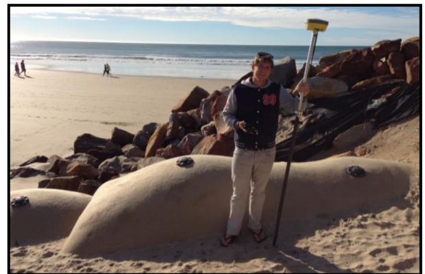
Figure 31: Textile sand bags placed on the artificial spit furthest from the Kromme River estuary mouth (Photo: Miller, 2014)
