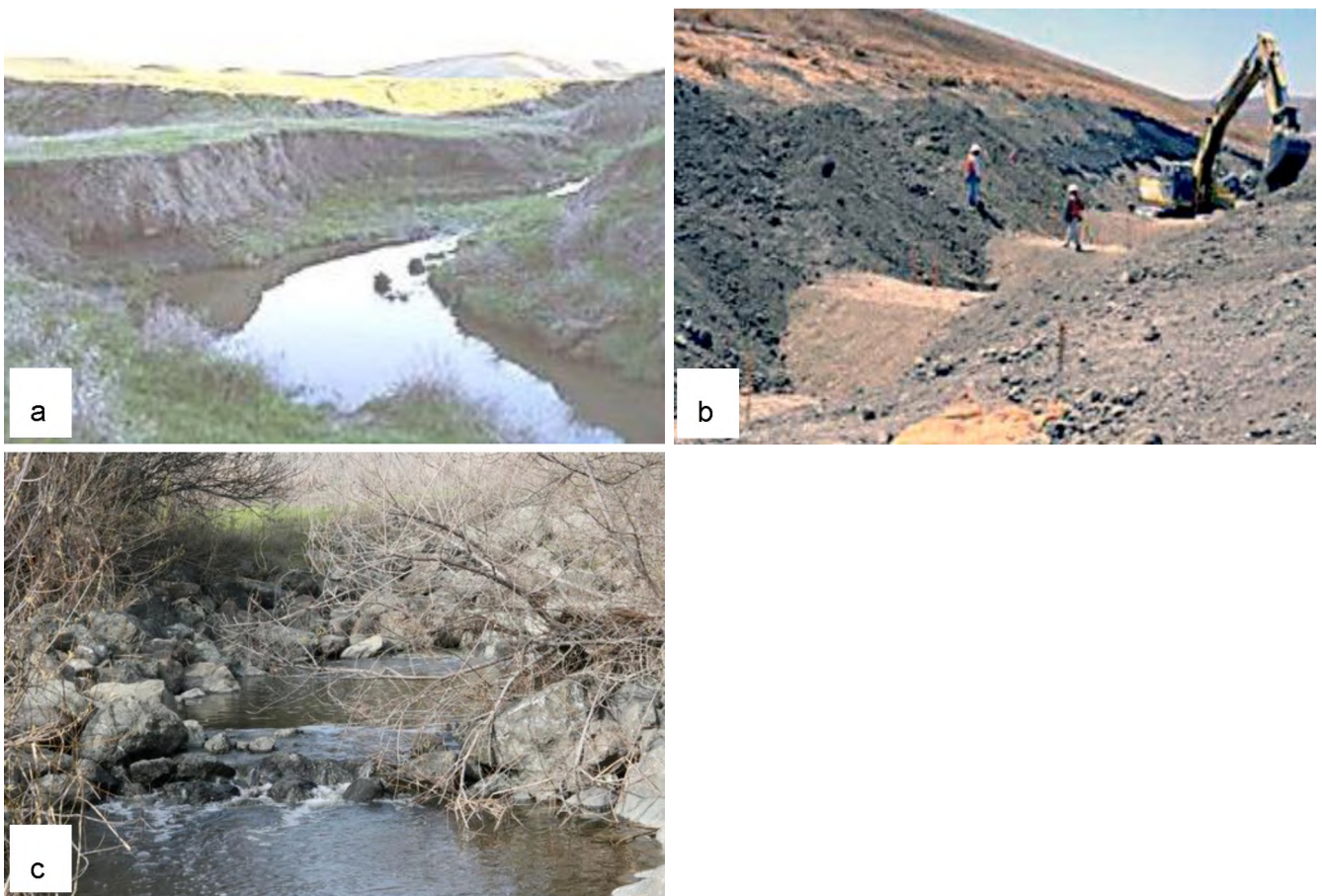
Plate 7.1: Rehabilitation of an incised channel reach (a), along East Alamo Creek in California. The re-shaped channel and floodplain and creation of artificial step-pool features are indicated (b), and the rehabilitated, relatively stable channel (c); (Photos by Jeff Haltiner).
