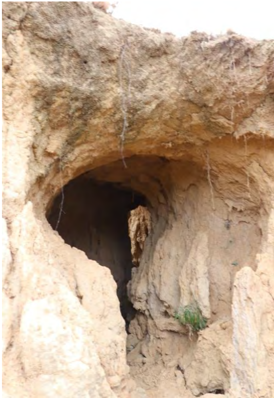
Figure 3.7 A photograph of a gully pipe network, a common feature of areas with duplex soils
