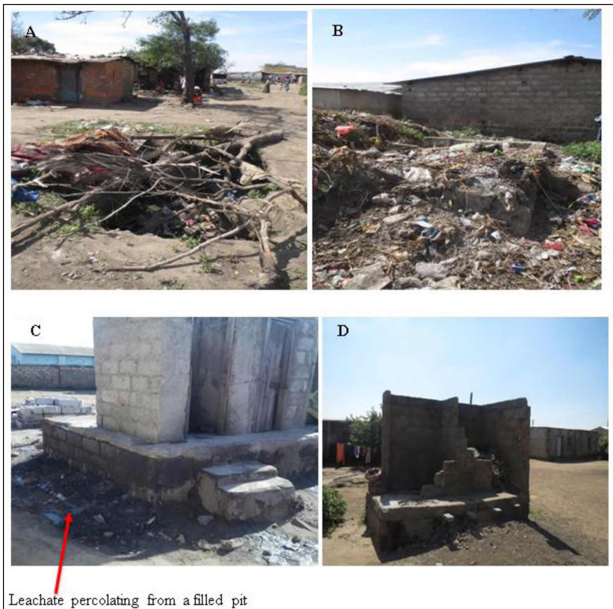
Figure 3.18: (A and B) Buried pit latrines (C and D) abandoned full pit latrine
