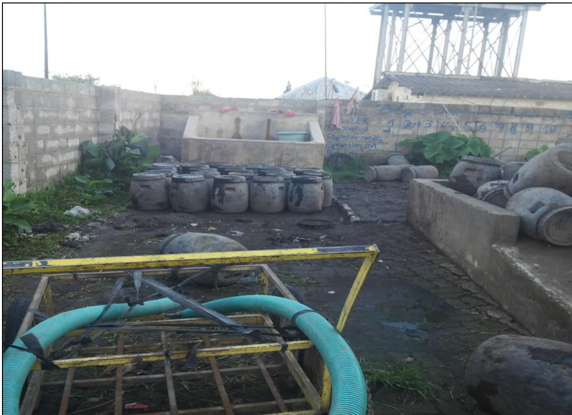
Figure 3.17: Barrels used for pit emptying by legal pit emptiers'
