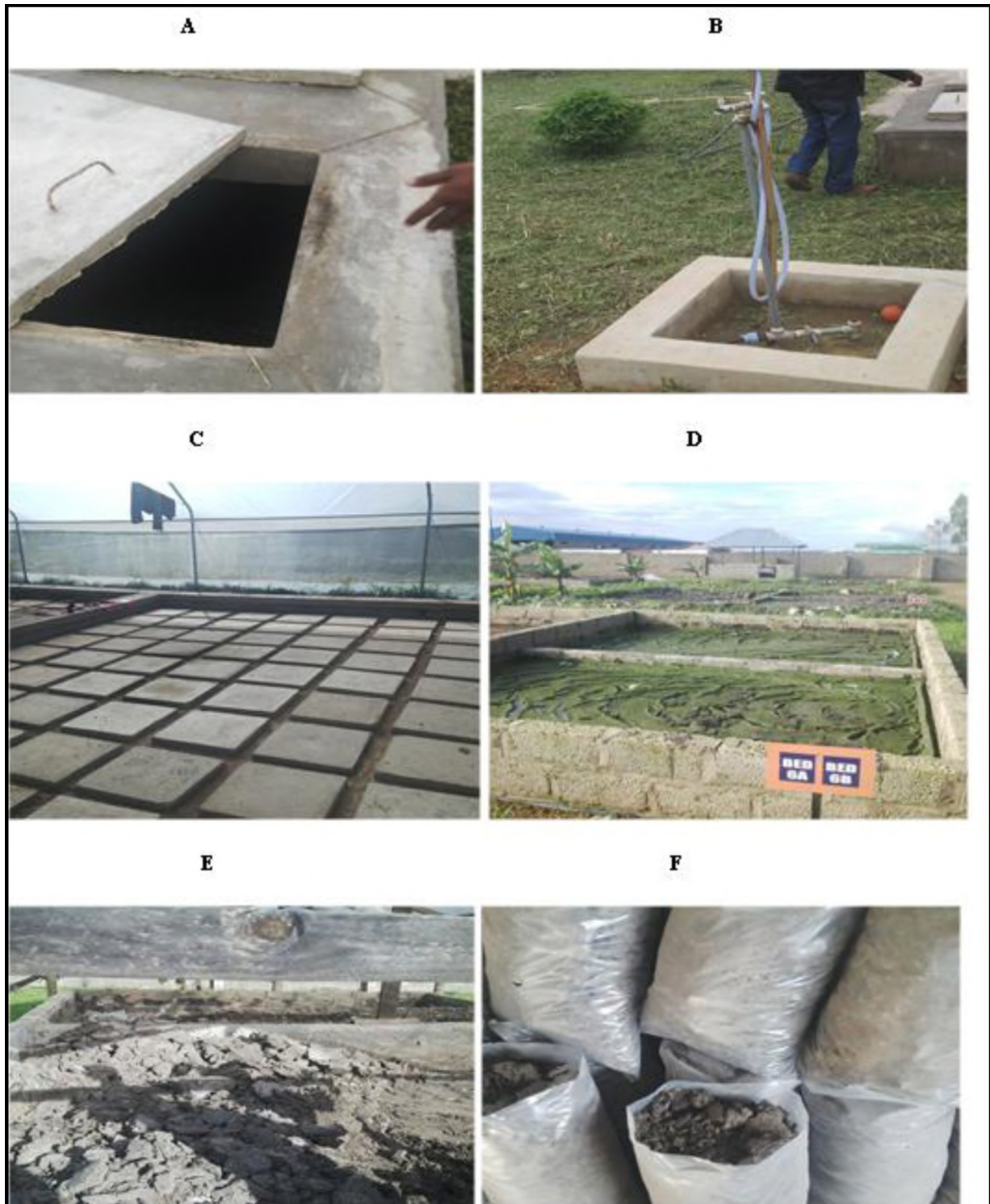
Figure 1.11: FSM stages (A) bio-digester, (B) gas pipe, (C) drying beds, (D) wet slurry in drying beds, (E) dried slurry and, (F) packaged dried slurry ready to sell
