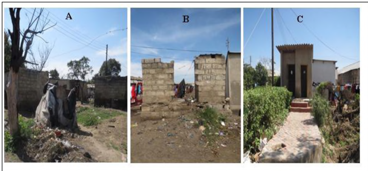
Figure 3.9: Contrast in sanitation technologies within Kanyama and Chazanga. (A) Unimproved pit latrine with a superstructure made from plastics, (B) unimproved pit latrines also used as a bathroom in Kanyama and (C), a VIP latrine in Chazanga
