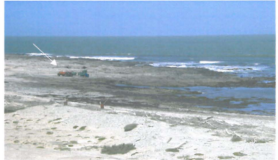
Plate 5.6: Shore-based mining diamond operation (white arrow) along the 'surf zone' of the Namaqualand coastline.
