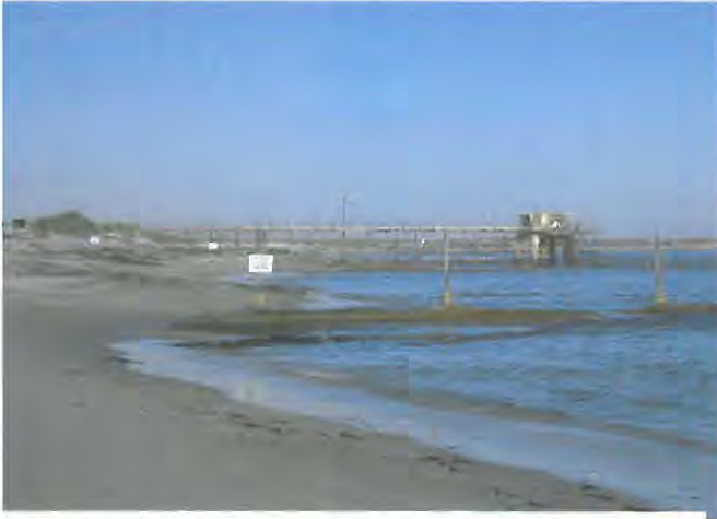
Plate 5.9: Pump station no. 7 (i.e. Oubeep) located south to Port Nolloth.
