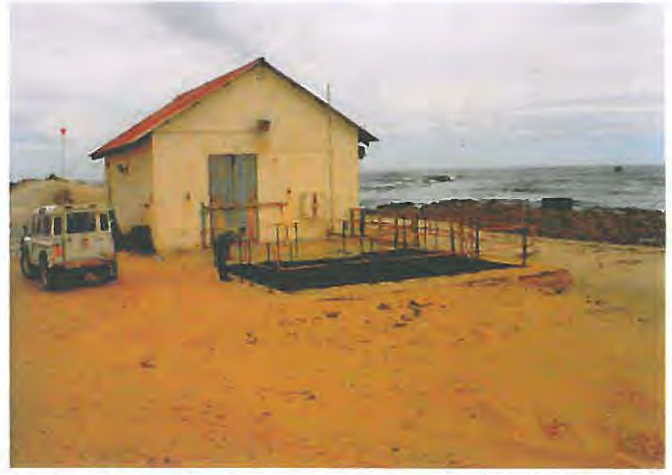
Plate 5.10: Pump station no. 10 (i.e. AK3) located north of Kleinsee.
