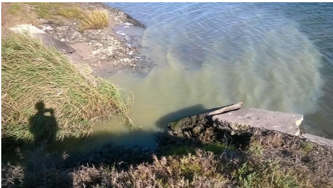
Figure 4.1: Images showing industrial effluent coming through from Markman industries. Top image shows the canal in which effluent is channelled towards the estuary and the bottom image, industrial effluent is discharged into the Swartkops (Source, Glen Vembo).
