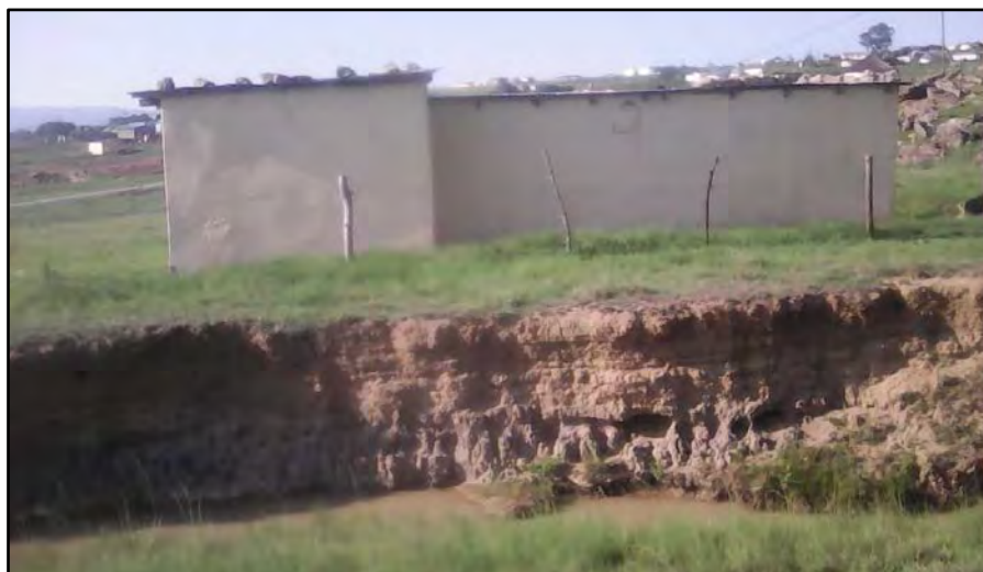
Figure 5.30. A house threatened by an erosion gully. Christopher Matsoso, a community liaison officer for the Tsitsa Project, took the photo in February 2020.
