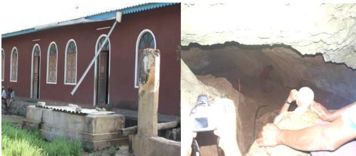
Plate 4.2: (Left) Local method for harvesting rain in one of the mosques in Kiuyu Mbuyuni, Pemba. (Right) Black pipe with pump used to draw water from one of the coral caves in Matemwe, Unguja
