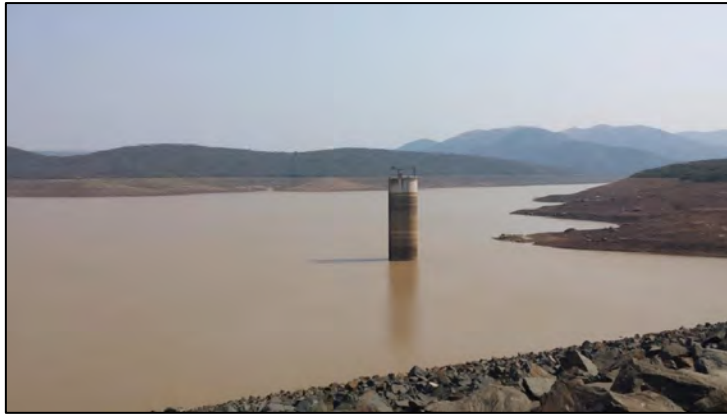
Figure 3: The Goedertrouw Dam that supplies water to Richards Bay and surrounding areas at a level of 16% in 2016 (Photo: Alex McNamara, 2016)
