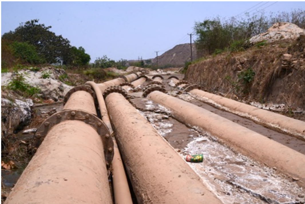
Fig.vi. Nchanga Mine Pipeline in Chingola, Zambia (2017), photograph by Stary Mwaba.
