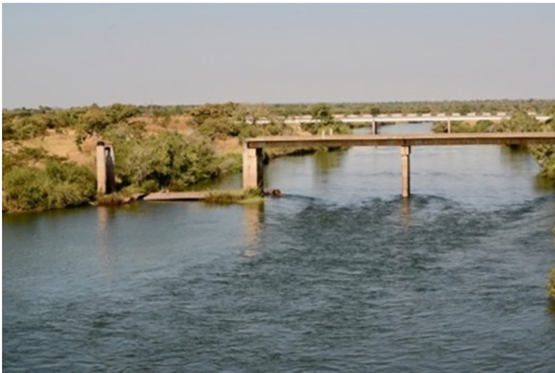
Fig. 2.7. Old Chambeshi Bridge that was bombed, Chambeshi, Zambia (2017), photograph by Sary Mwaba.
