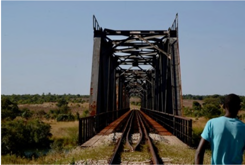
Fig. 2.6. Detail of Uhuru railway or Freedom Railway Bridge, Chambeshi, Zambia (2017), photograph by Sary Mwaba.
