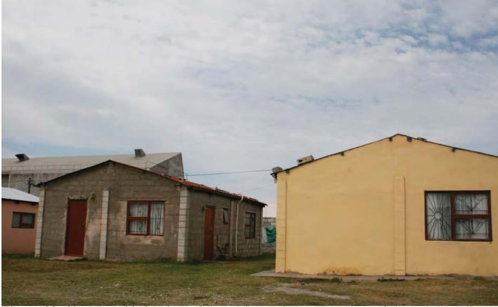
Figure 28: Sippel, E. 2010. View of the Red Location Museum's roof through the adjacent houses. [Photograph] (Reproduced with permission from the Red Location Museum).
