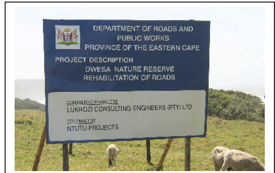
Plate 14 – A road rehabilitation project.
