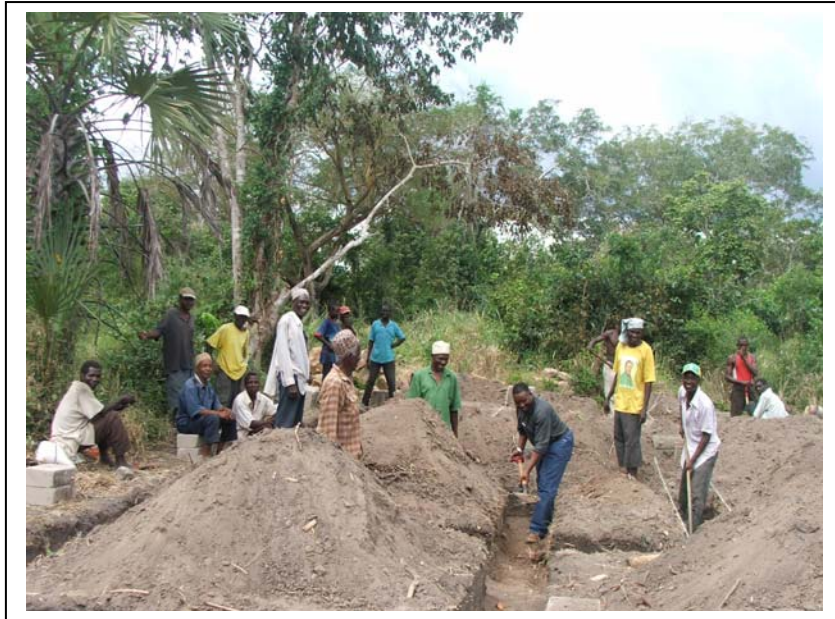
Photograph 16. School committee members and other community members building the teachers' house
