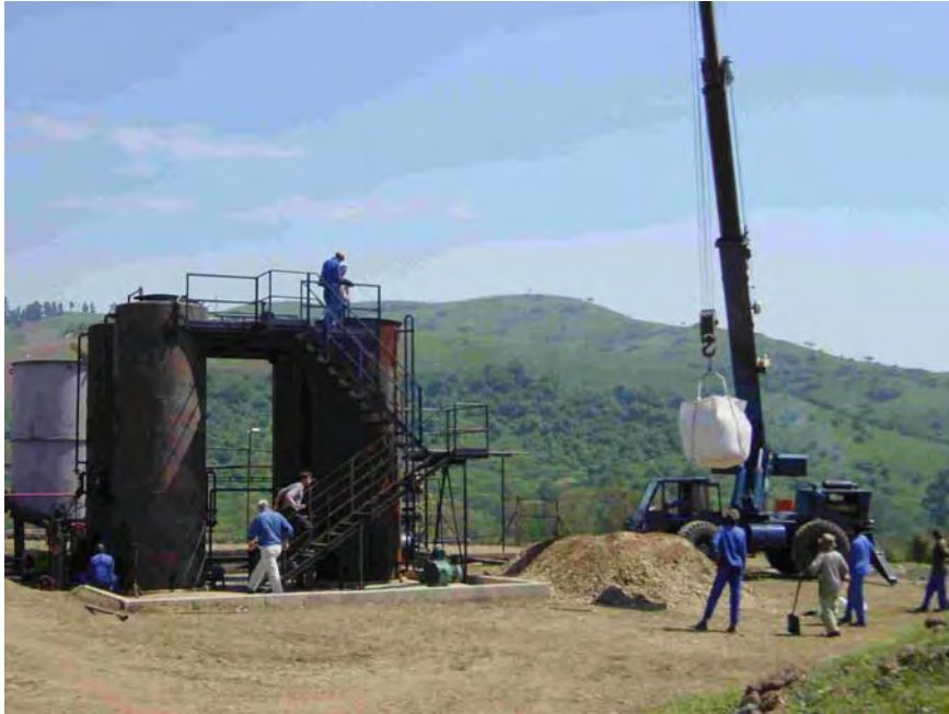
Figure 6.1 The reactor was packed with the wood chips by employing a loading bag and crane.
