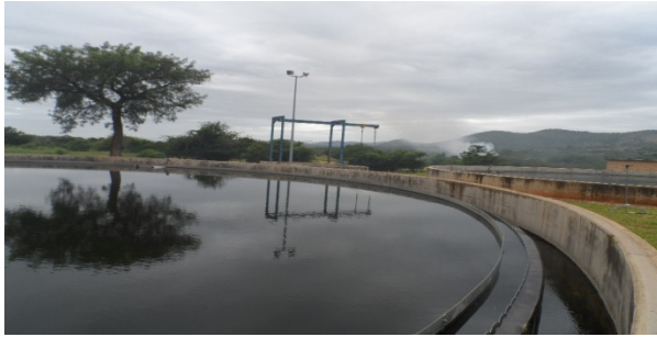
c. Clarifiers clear of algal growth
