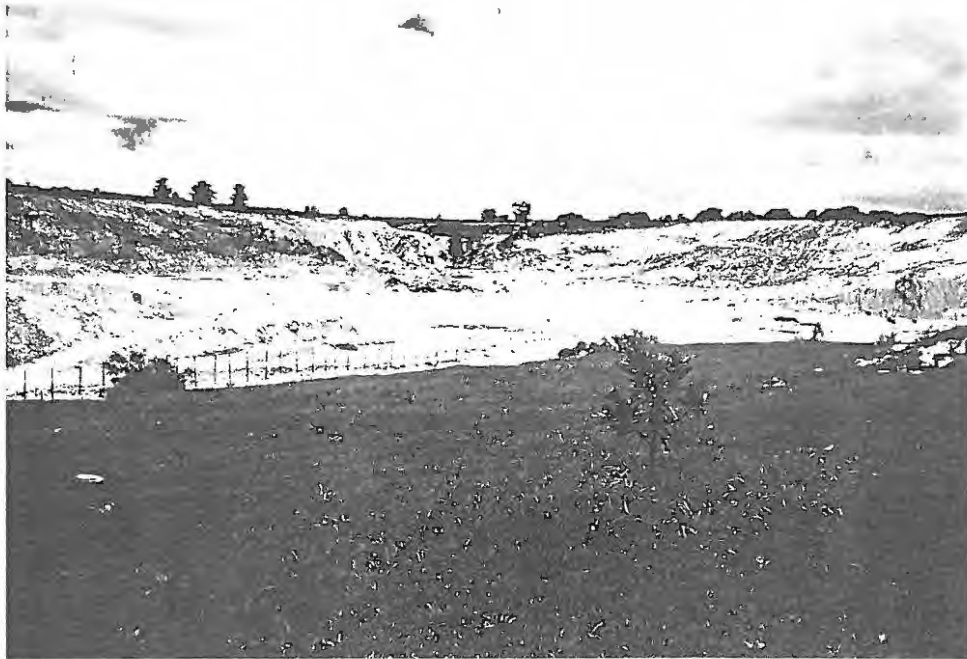
Photograph 2. The Rehabilitated Site.
