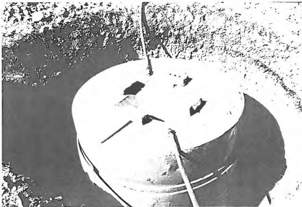
Photograph 5. Initial Testing of the Gasometer.
