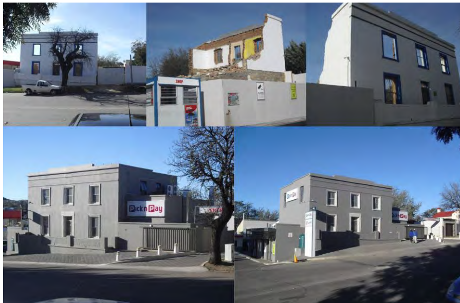
Figure 5.13: Pick n Pay in Bathurst Street before and after construction (Grahamstown Eye, 2019).
