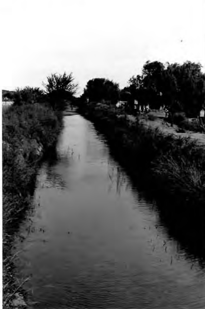
PLATE 2. The Middleton Canal - An example of an unlined earth canal.
