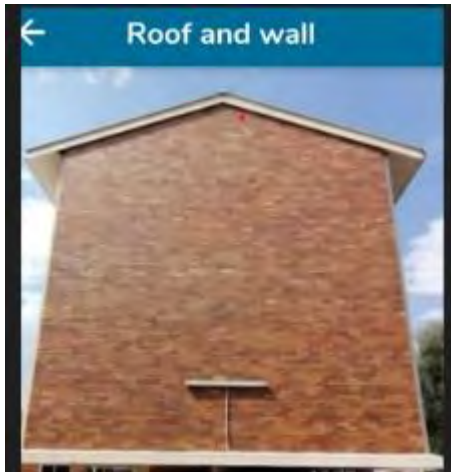
Figure 4.19: school wall and roof
