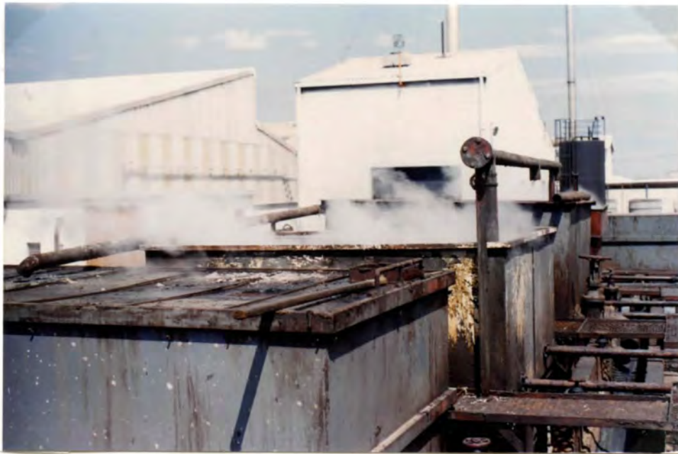
Plate 2.4. The hydrolysis reaction in progress.
