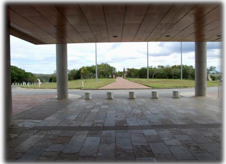
Fig.13. 1820 Settlers National Monument: Phase One, Ground Floor. Photograph: Simone Heymans
