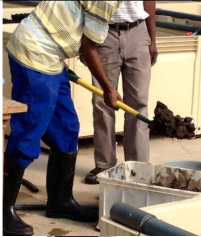
Removing and replacing sediment
