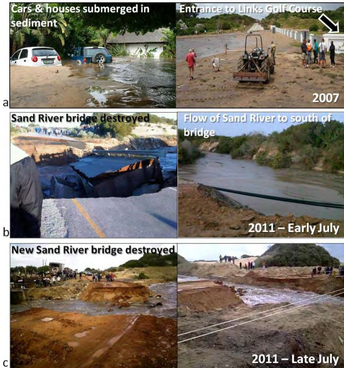
Figure 6-11 (a, b & c): The destruction caused as a result of floods and/or debris flows largely related to extreme and intense rainfall events. a: massive flood event over Links Golf Course 2007, b & c: debris flows destroying the Sand River Bridge across the R303 in 2011.
