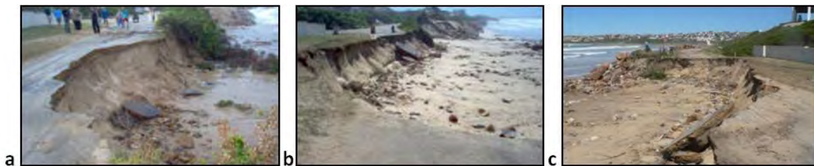
Figure 1-3 (a, b & c): Erosion of Ralph Road along the St. Francis Bay shoreline. Photographs 2a and 2b were taken 24 hours apart in March 2007, during which time the width of the road was reduced by erosion.
