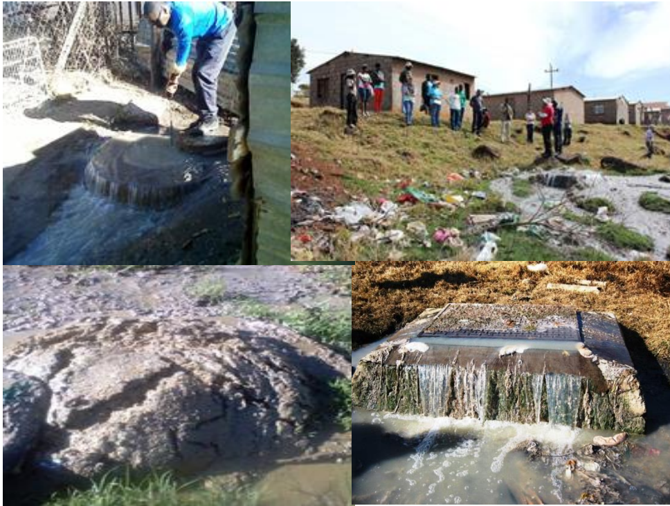
Figure 3: A collage of photos of spilling sewerage manholes also featuring an illegal dumpsite. Raw sewage runs directly into the uMthinzima stream (Photos: L. Taylor, 2013).
