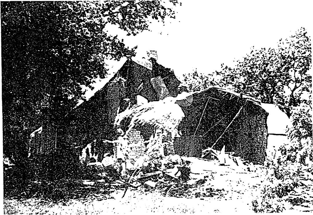
Figure 4.4. Damage to a building caused by the Ceres/Tulbagh earthquake of September 1969 (after Keyser, 1974).
