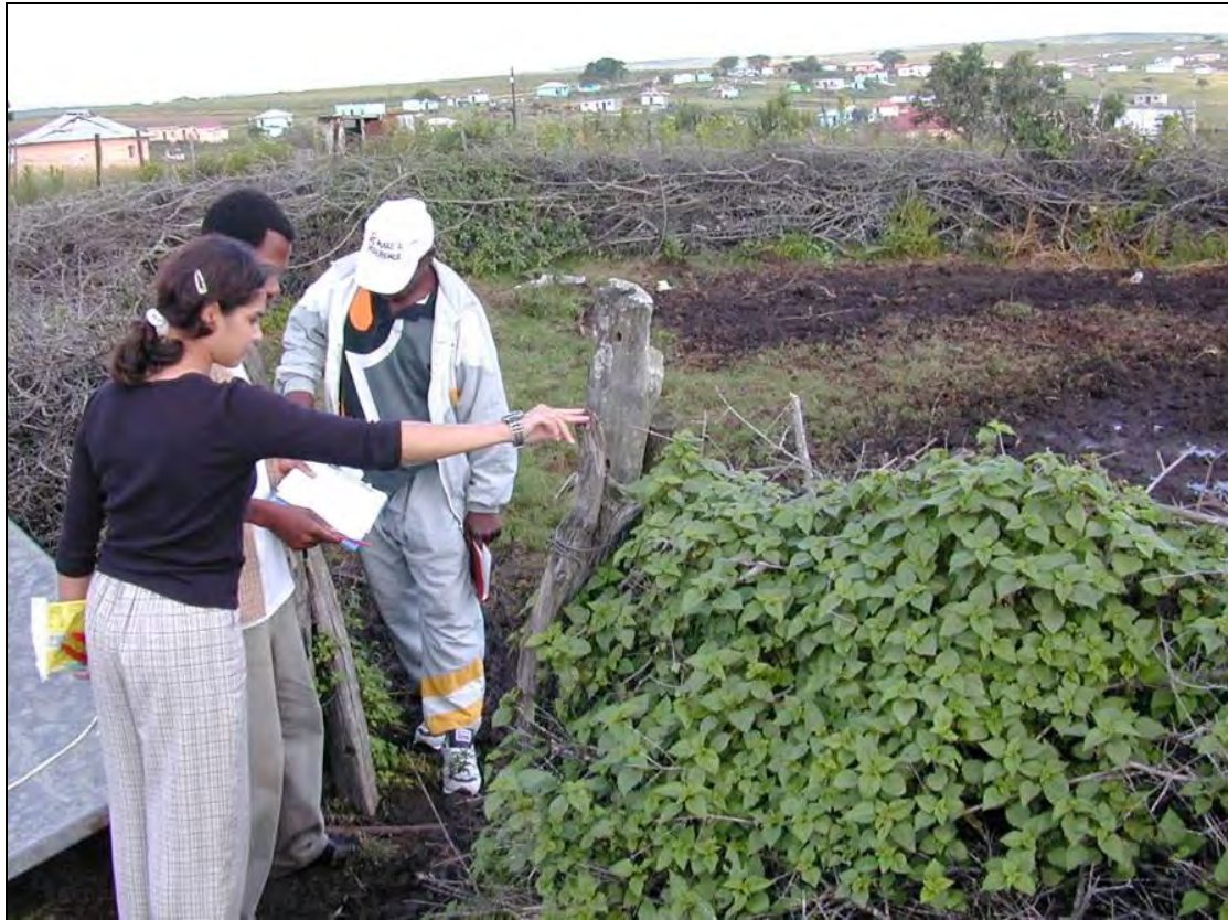
Figure 1.2: Traditional Xhosa kraal, constructed from brushwood and kraal posts
