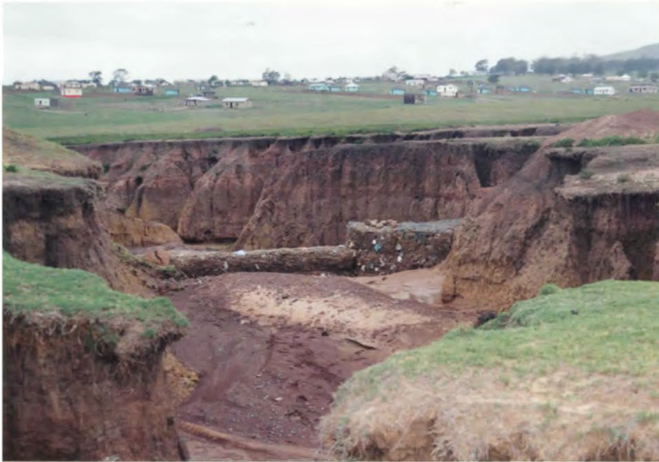
Plate 24 Ross Mission Area - The effect of anti-erosion walls is evident
