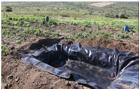
An example of a completed homestead pond for storing rainwater from crop production.
