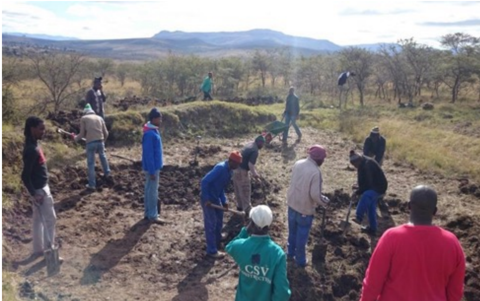
Figure 4.21: College students with workers providing manual labour in the productive demonstration development
