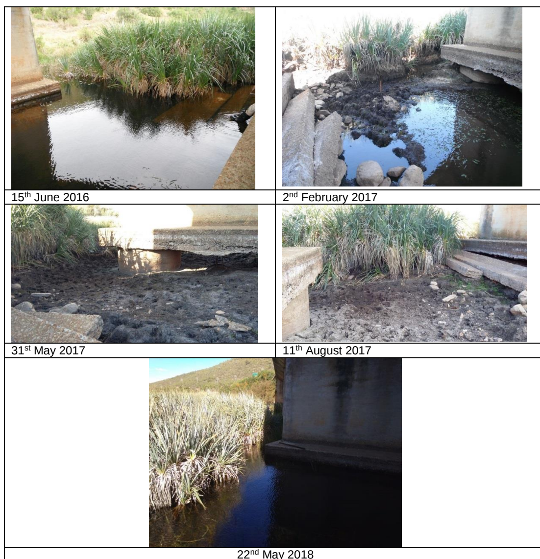
Figure 4.4. Illustration of the variation in water levels at the top of the Kompanjiesdrif wetland (underneath the R62 bridge: -33.878420°, 24.053210°). A particularly dry period was experienced in the catchment between February and August 2017.
