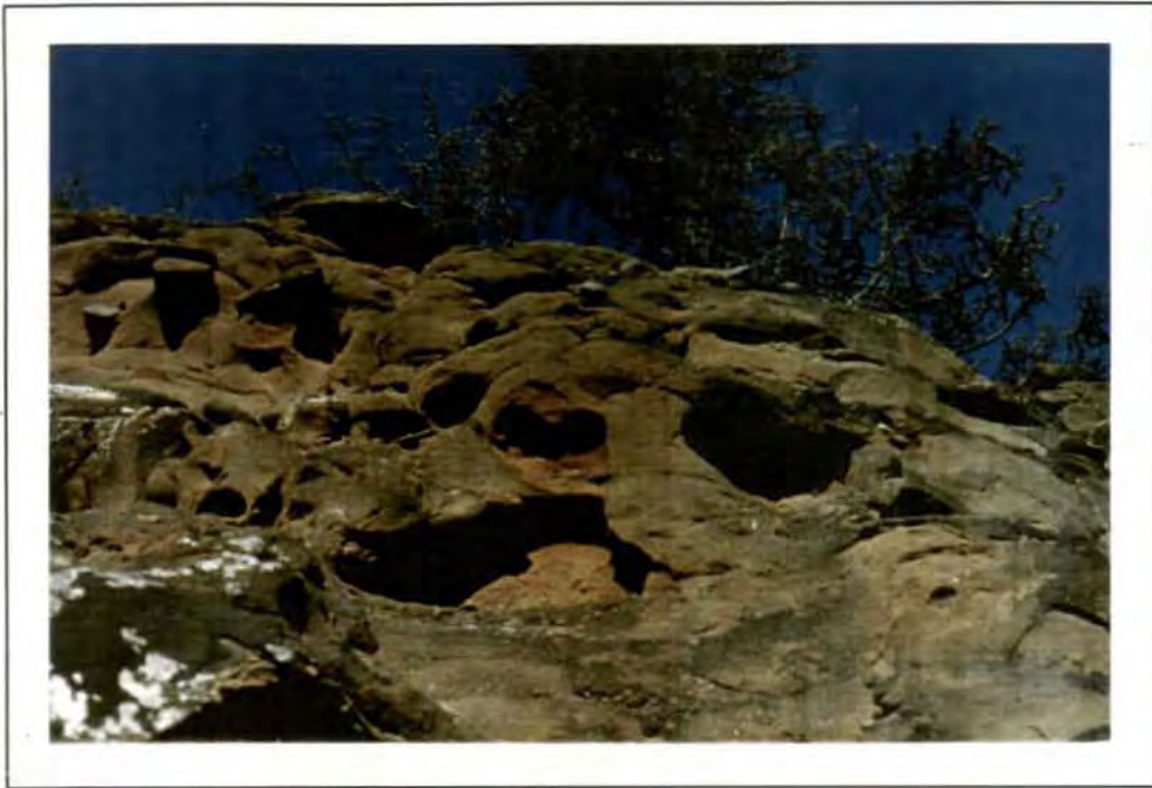
Figure 14. Pitted sandstones exposed in section D (Appendix 1) due to preferential weathering.
