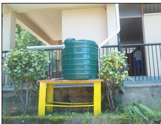
Photograph 4.31 Phase One of the Rainwater Harvesting project
