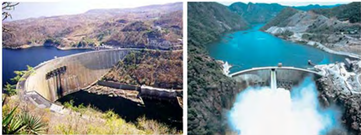
Figure 3.10 Kariba Dam (left) and Cahora Bassa Dam (right: source: Bourgeois et al., 2003)
