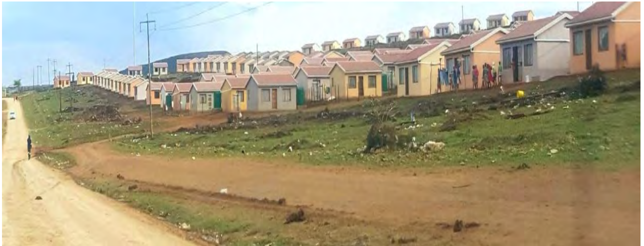
Figure 5.2: Example of how the houses in low-cost housing areas are arranged and the spacing between households.
