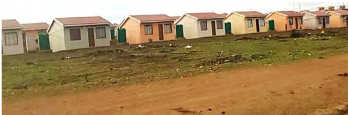
Figure 1.1: A recently developed low-cost housing area in the Eastern Cape, 3 km from the CBD exhibiting a spatial pattern of apartheid (Picture taken by researcher, 2017).
