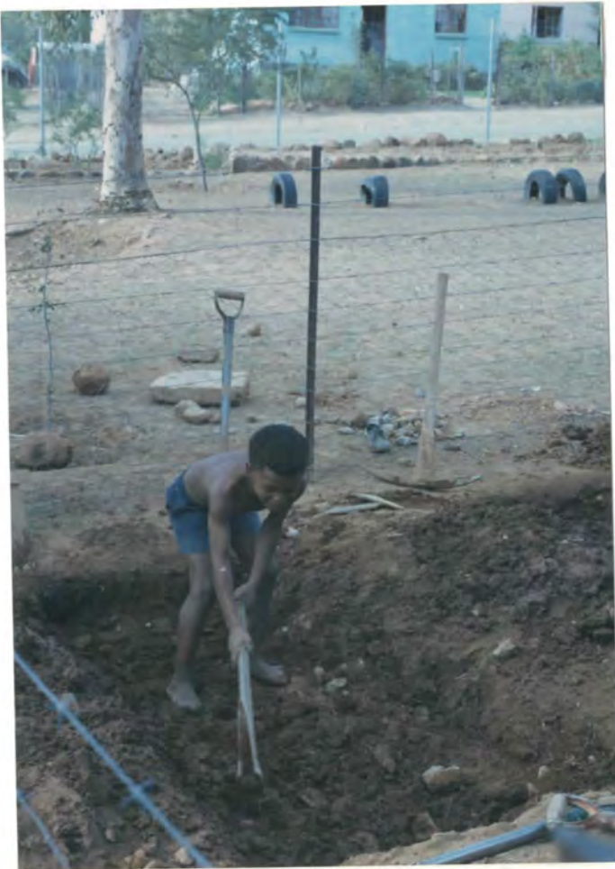
FIGURE 5.2: PREPARING THE TRENCH GARDEN
