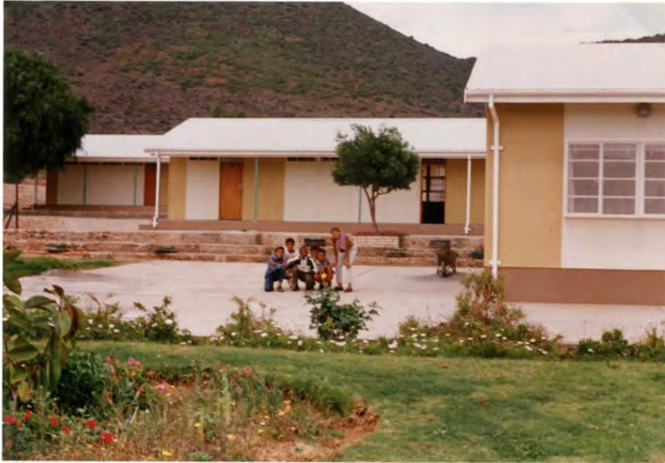
FIGURE 1.4: A SECTION OF THE RYNEVELD PRIMÊRESKOOL IN KROONVALE, GRAAFF-REINET.
