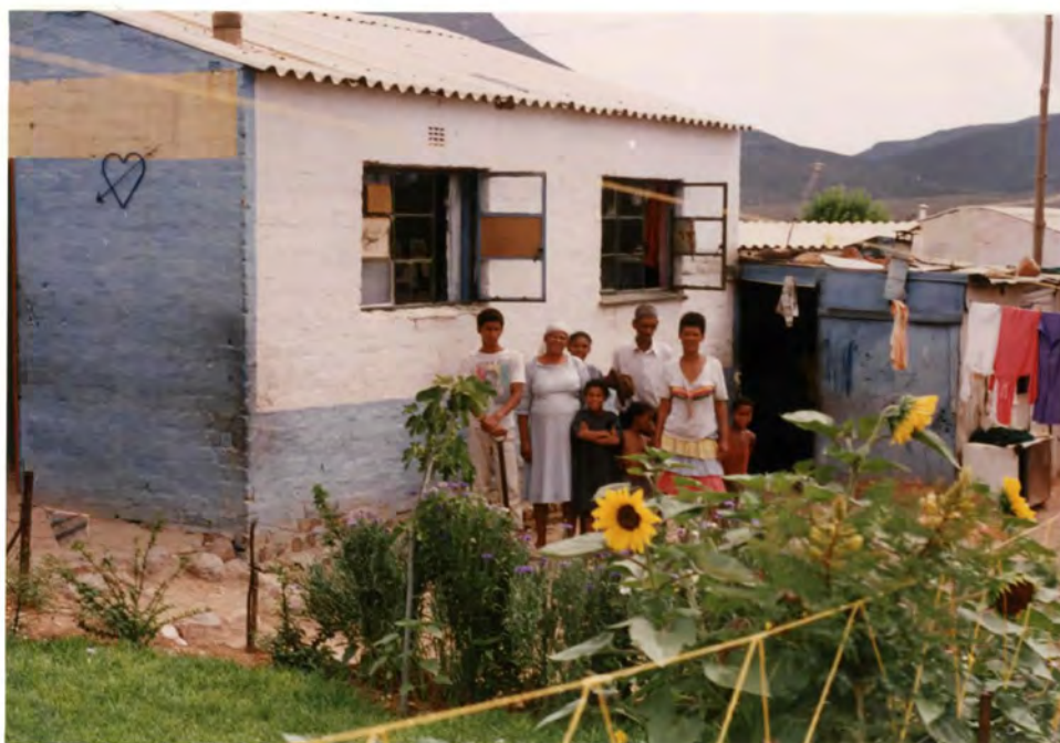
FIGURE 1.1: A TYPICAL 2-ROOMED SEMI-DETACHED HOUSE IN KROONVALE, GRAAFF-REINET.
