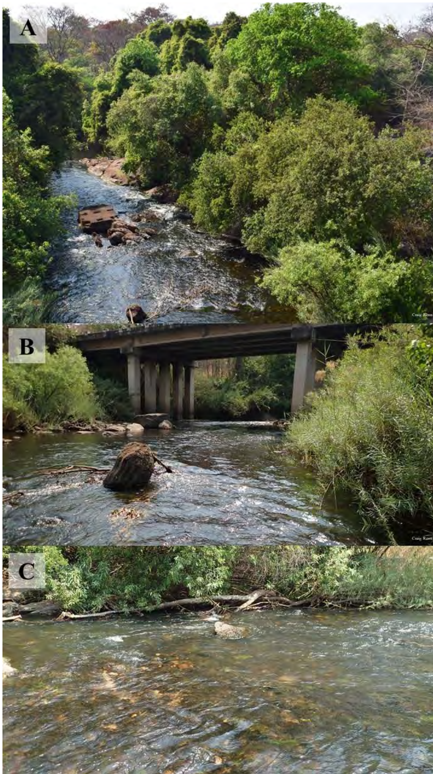
Figure 2.4 Kabompo Bridge site on T5 road, a headwater site on the Kabompo River, Zambia, as seen from: A) above, B) upstream, and C) downstream.
