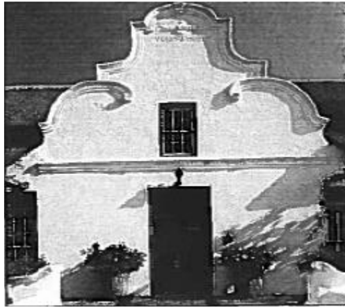
Fig. 16: Inland gable- is of the period 1750- 75. Here the mouldings curve forward onto the gable face (Source: Simmons 2000: 11)
