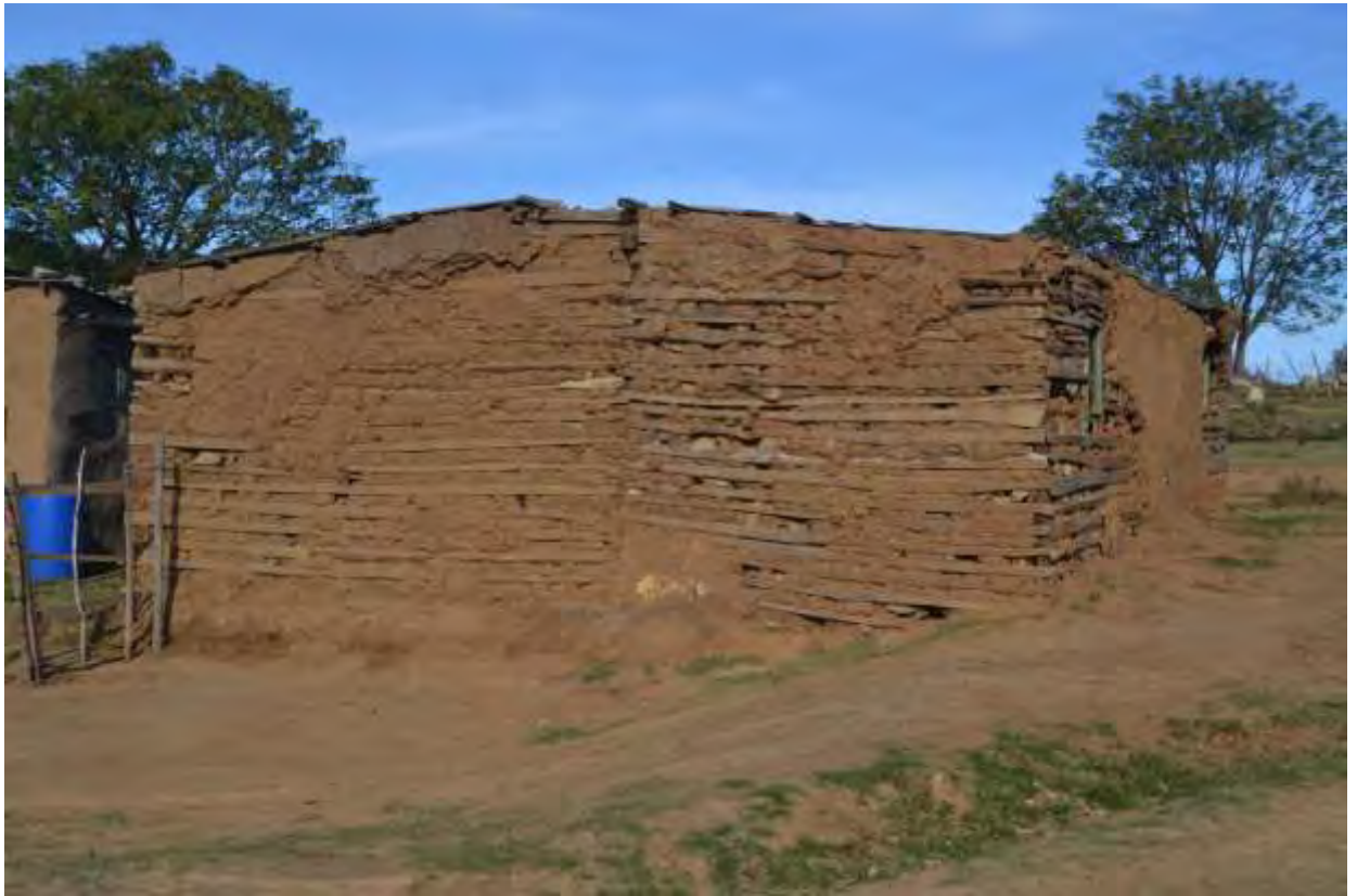
Fairbairn household showing the natural resources used to build it e.g. mud and sticks
