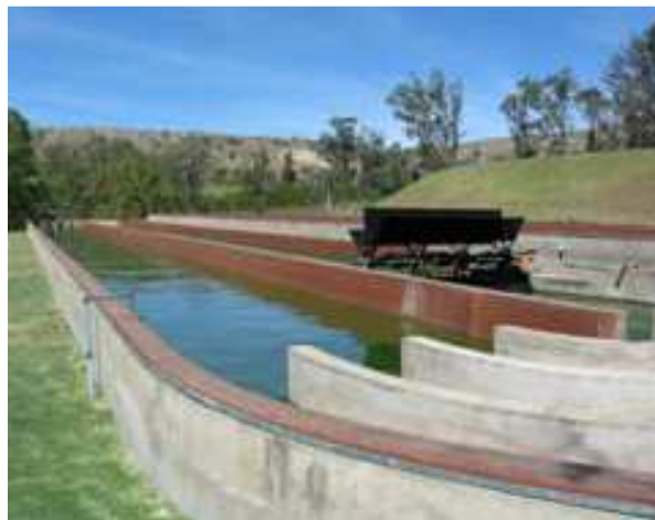
Figure 2-1: The second HRAP in series in the IAPS at the municipal WWTP in Grahamstown, from which sampling took place.
