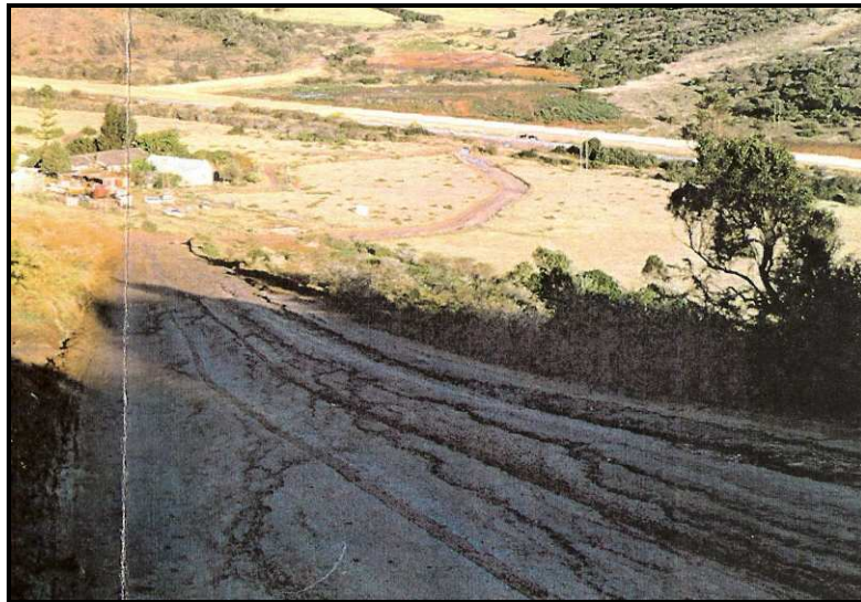
Figure 2.11: Access road to a Department of Roads and Transport quarry showing the development of significant rill erosion – Eastern cape (DME archives).
