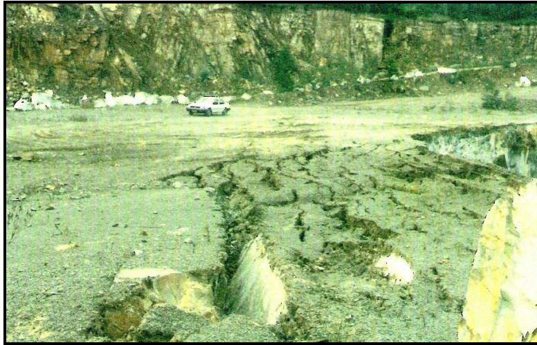
Figure 2.12: Hard rock quarry showing rock face slumping – Eastern Cape (DME archives).
