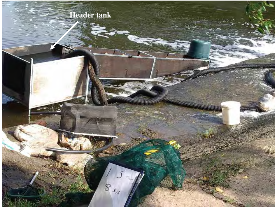
Plate 2.6: Sloping Baffle Fishway position 2, below lower apron with water diverted towards entrance.
