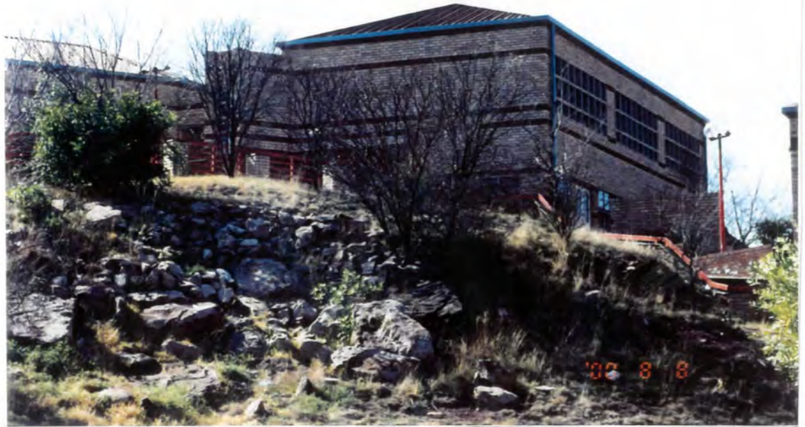
Figure 2a: The college administration block and lecture rooms
