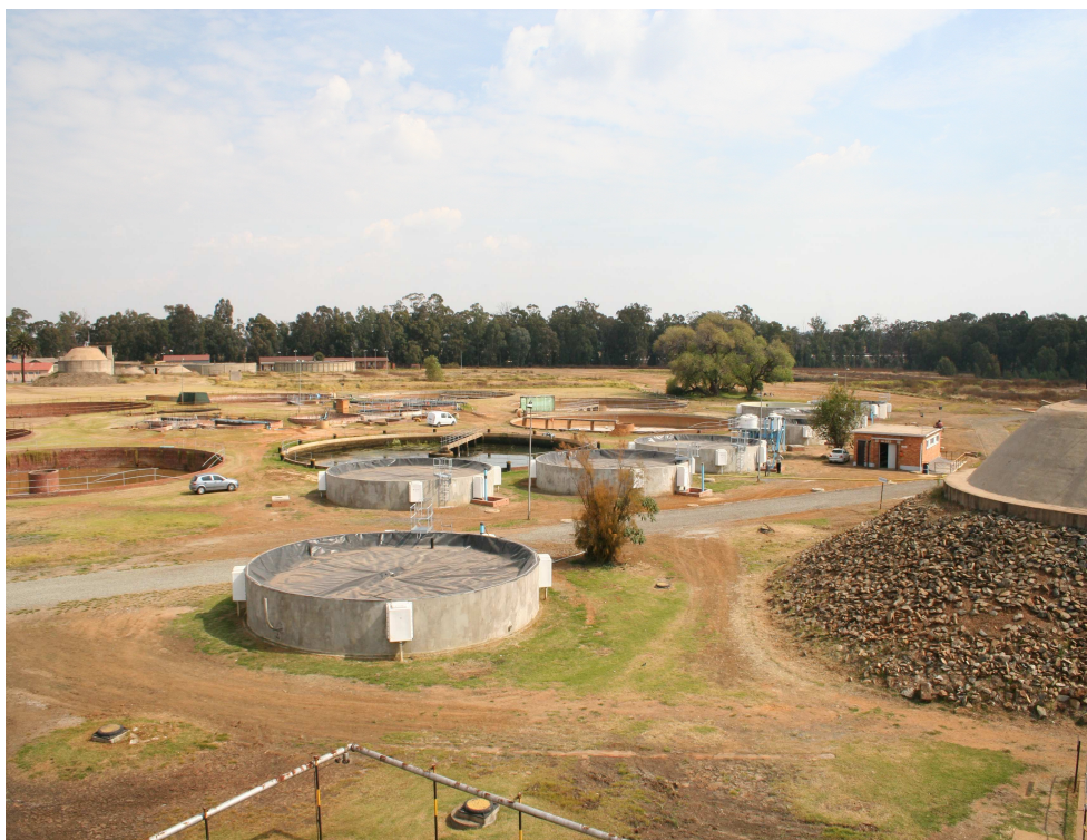
Figure 8.2 Photograph of the full-scale Rhodes BioSURE Process plant showing sealed individual unit upflow Recycling Sludge Bed Reactor (RSBR) modules and mine water feed tanks, clarifiers and final effluent dam in background.
