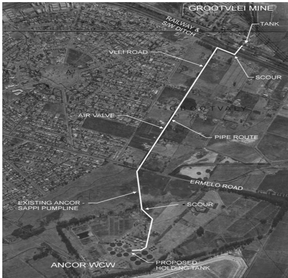
Figure 4.5 Photograph showing pipeline route between Grootvlei Mine and Ancor Works (Springs) through which mine water was supplied to the Technical-scale Multi-stage Reactor.
