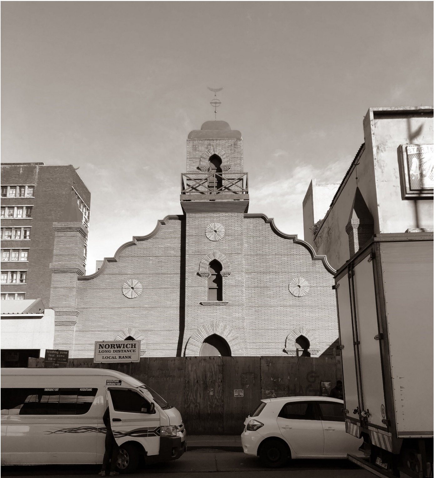
Figure (23): The external façade of the Strand Street Mosque (source: author)
