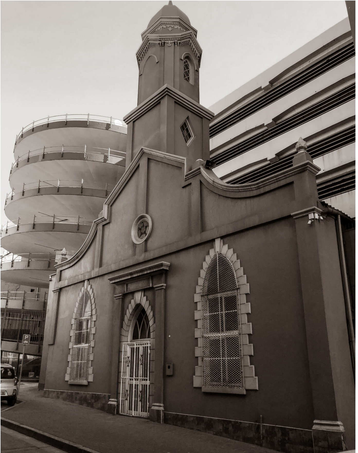
Figure (6): The external façade of the GSM (source: author)
