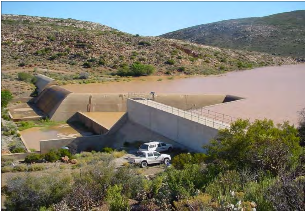
Figure A3.9: The Prinsriver Dam, illustrating the topography and vegetation of the lower part of the catchment.
