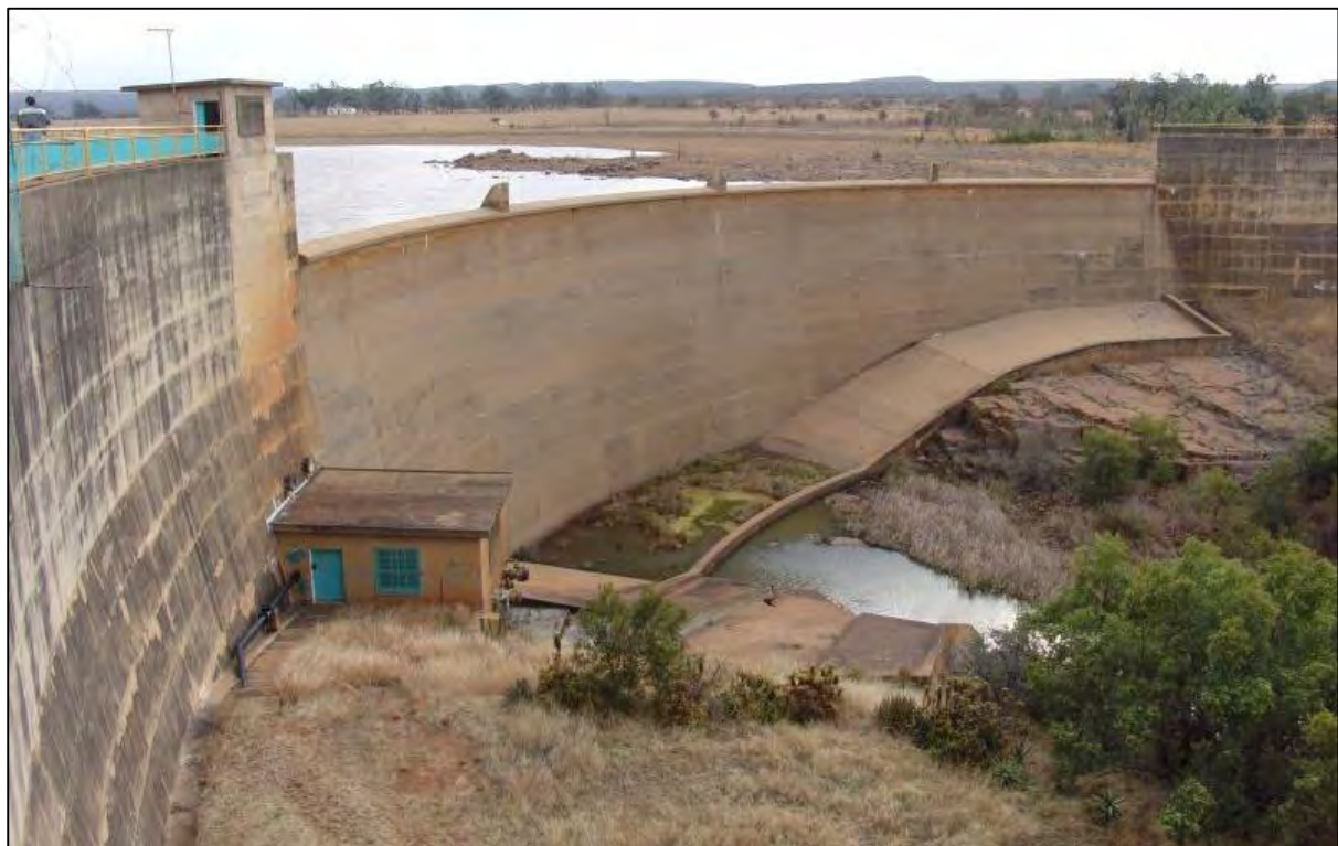
Figure A3.16: Image showing the Koster Dam.
