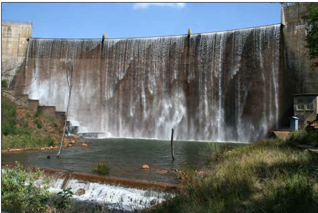
Figure A3.18: Image showing the Buffelspoort Dam.
