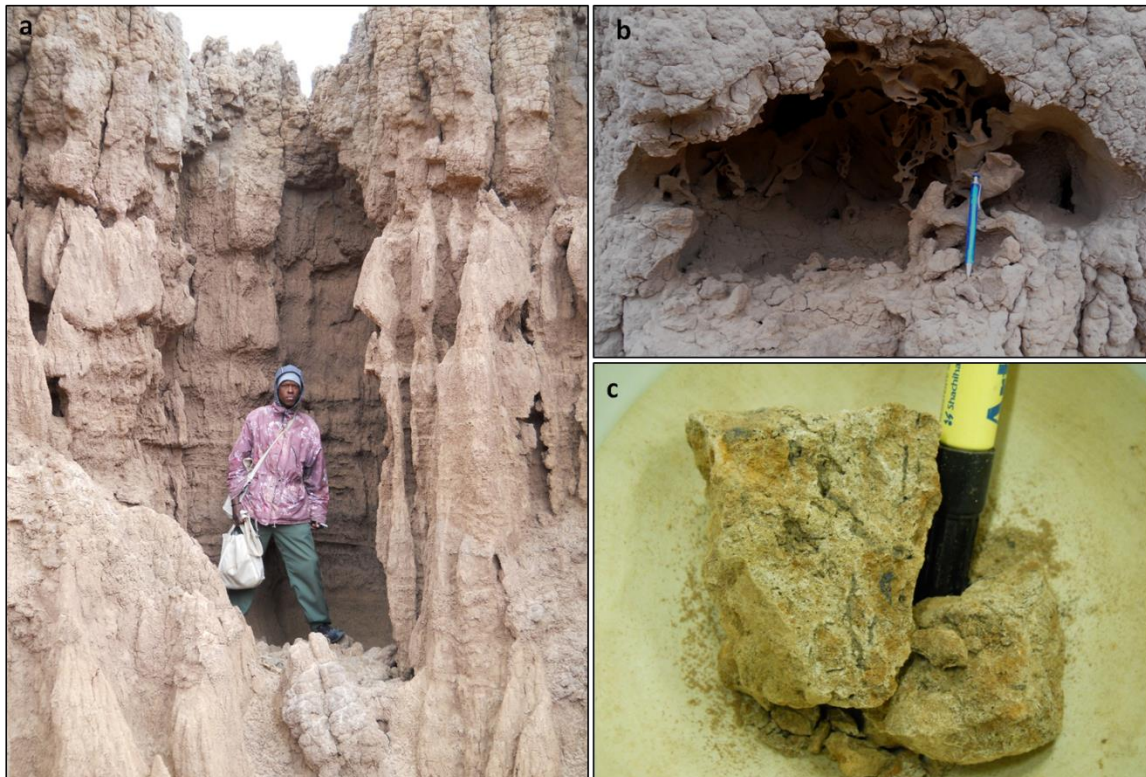
Figure 3.13: Associated erosion features in Taung sub-catchment (a: sidewall collapse b: cavities c: mottling).
