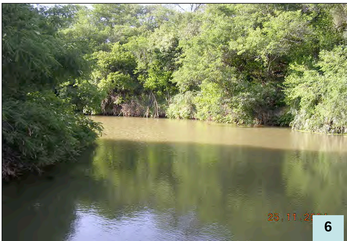
Figure A.6 Warden's Weir (Lower Kat).
