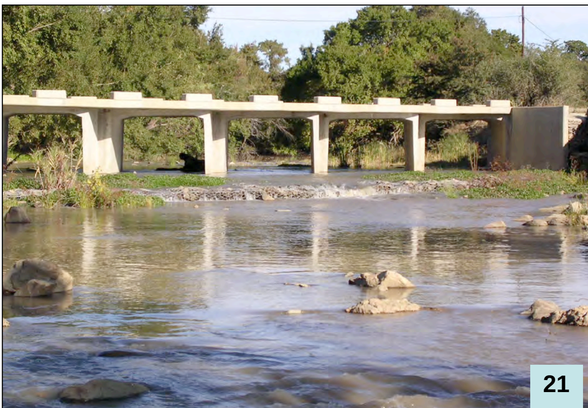
Figure A.20 Fairbairn Bridge (Upper Kat).
