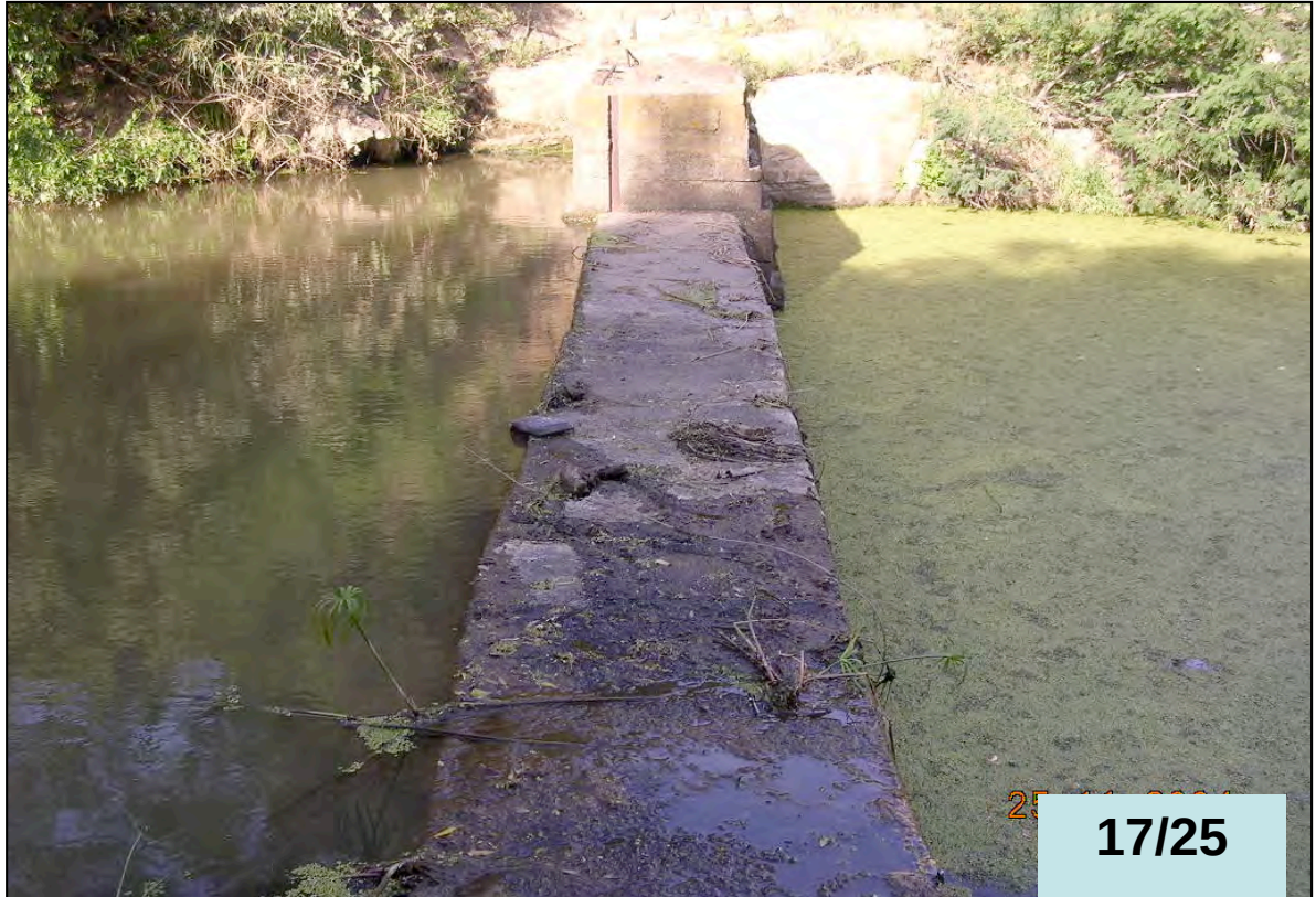
Figure A.24 Wardens Weir (Lower Kat).
