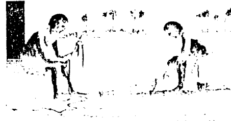
Two men are laying out a square on the ground by using a rope.
