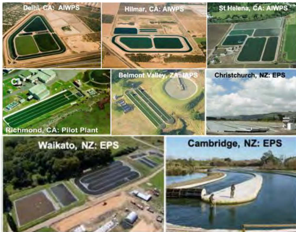
Figure 1:3: Examples of AIWPS and similar systems located in the USA, South Africa, and New Zealand. CA = California, NZ = New Zealand, ZA = South Africa. AIWPS = Algal Integrated Wastewater Pond System, IAPS = Integrated Algal Pond System, EPS = Enhanced Pond System. AIWPS has been implemented at pilot, demonstration, and full commercial scale.
